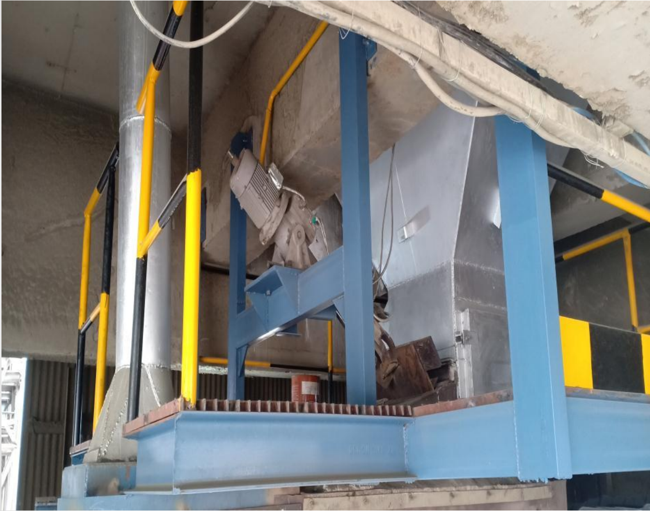
NEWLY INSTALLED IN-HOUSE FLAP GATE WITH OLD LINEAR ACTUATOR
