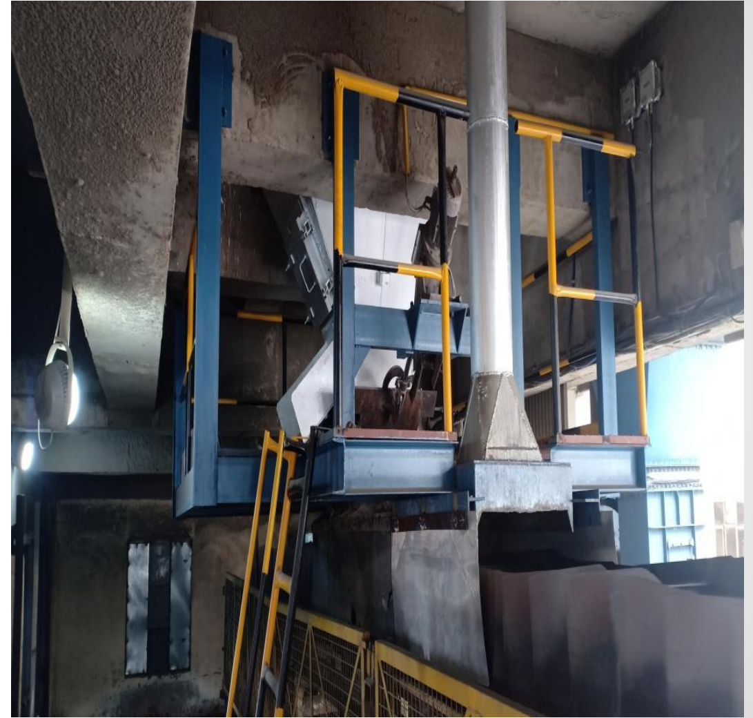
NEWLY INSTALLED IN-HOUSE FLAP GATE WITH OLD LINEAR ACTUATOR
